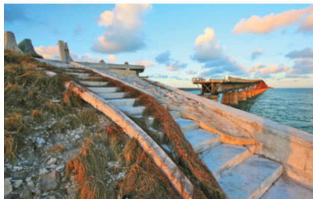
Remains of steps to the original bridge and railway at Bahia Honda. Photo credit Eddie Green
